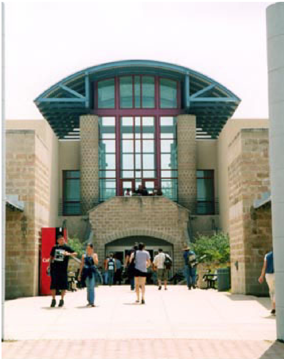
The two-story General Education Building in the center of the main campus houses classrooms and faculty offices.
