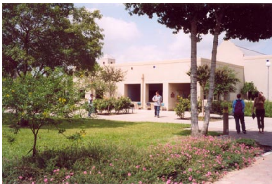
The Student Center is being expanded and is scheduled to be completed in 2005.
