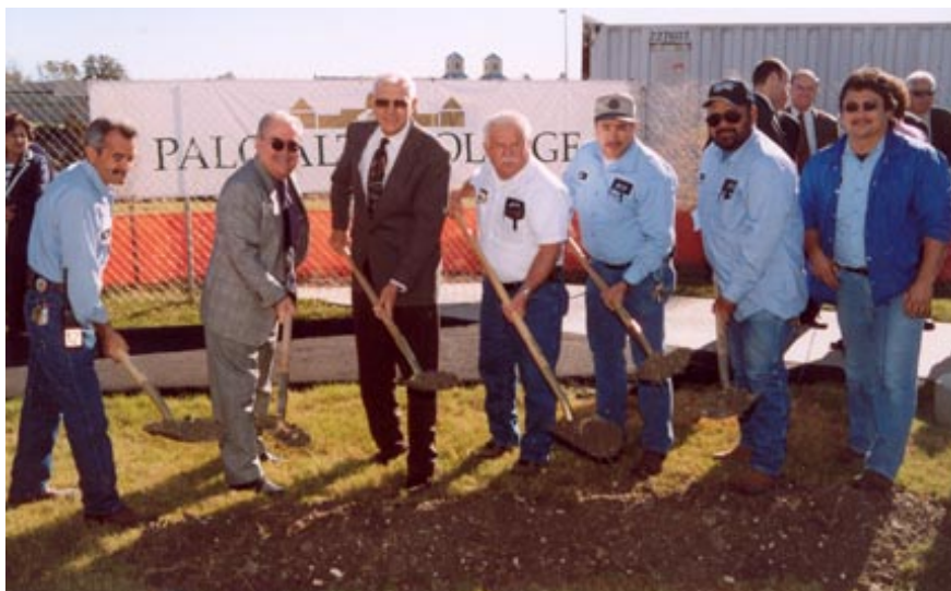
Facilities staff members, who are key to providing a safe and beautiful campus, celebrate the start of another campus building.
