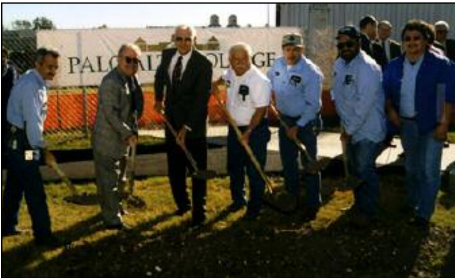
Facilities staff members, who will help maintain the new building, help break ground for the Applied Science and Technology Center.
